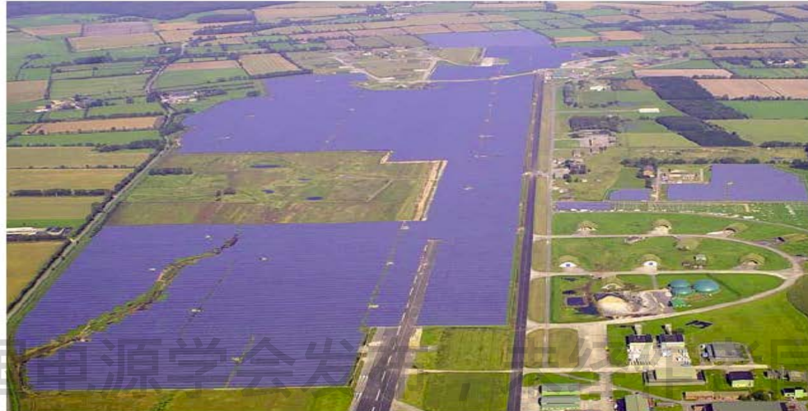
Figure 2. Aerial view of Eggebek solar plant. Courtesy of Möhring Energie
